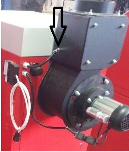
Figure 15. Placing the probe
